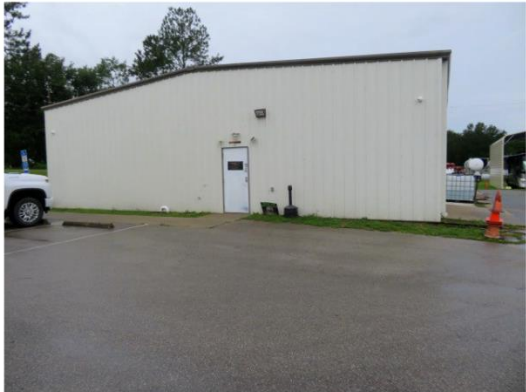
East building side
