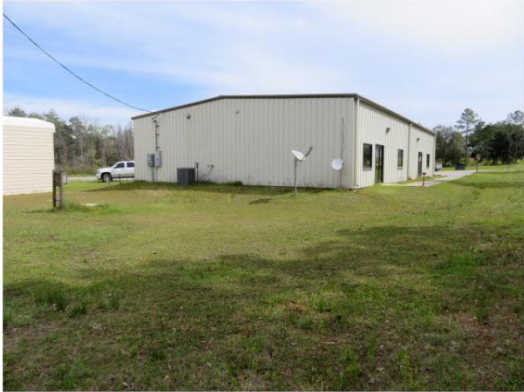
West side view
