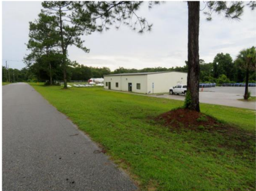
South side front view
