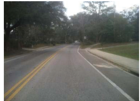
The beginning of the urban section and end of paved shoulders on US 90, west of downtown Monticello. This location could have a Share the Road or Bikes May Use Full Lane sign, as well as sharrow markings to help cyclists transition from the shoulder to sharing the travel lane.
