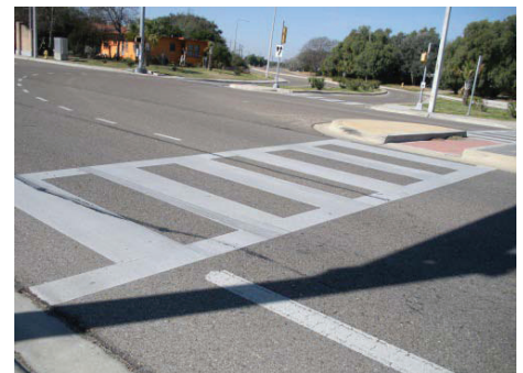
High-visibility ladder style crosswalk markings, Corpus Christi, TX.
