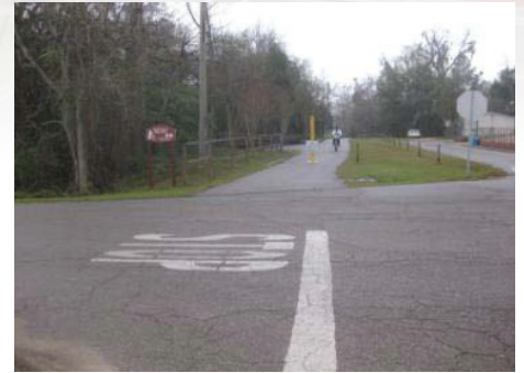
The Ike Anderson Trail ends at Rocky Branch Road. However, there is no crosswalk connecting the trail to the sidewalk that continues on the north side of the intersection. If one was added, the stop bar would need to be shifted back.
