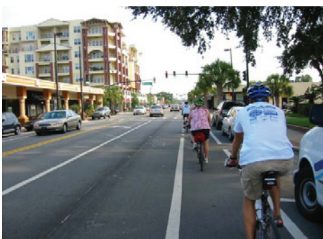
A "road diet" project converted Edgewater Drive in Orlando, FL from a 4-lane undivided roadway to 2-lanes with center turn lane and bicycle lanes.
