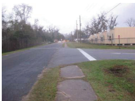
Sidewalks near the school are of substandard width, minimally separated from the roadway, and in poor condition. There is an unnecessary marked crosswalk across Rocky Branch Road, but no marked crosswalk across school driveway, as shown in the picture above.
