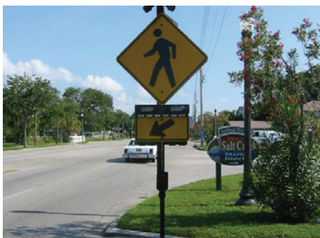
Closer view of the RRFBs mounted underneath the pedestrian warning sign.
