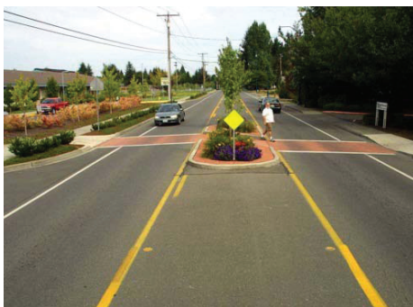
Example of median refuge island with angled crossing.
