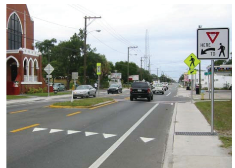
Midblock crosswalk with median island, advance yield lines, yield here to peds sign, and in-street pedestrian crossing sign, Tampa, FL.
