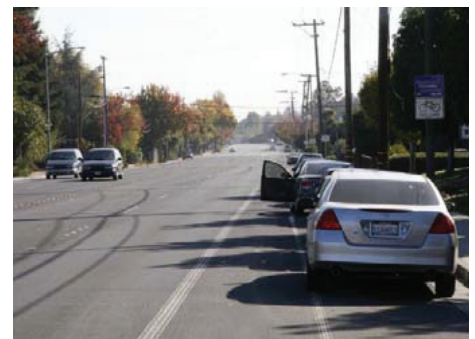
An example of a bike lane located within the “door zone” of the adjacent parallel parking lane.
