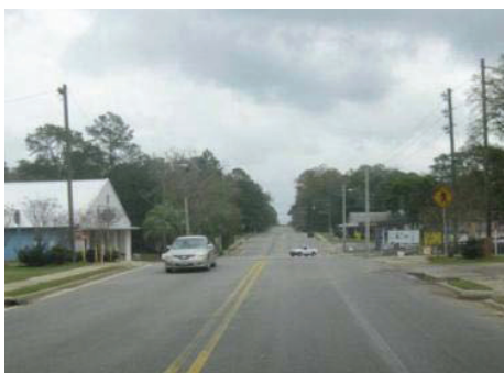
The trail crossing at US 90 is not very visible. There is an opportunity to improve signage, lighting, and potentially install a refuge island to facilitate crossing one direction and one lane at a time.
