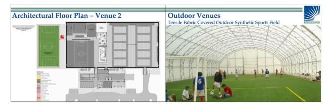
Adjacent to the air-supported structure is a tension fabric covered outdoor synthetic turf field. The turf field is  $200' \times 100'$  and provides a standard training field for long field sports such as soccer, lacrosse, football, and field hockey. This amenity will provide year-round space for youth and adult leagues, training, camps, and clinics.
