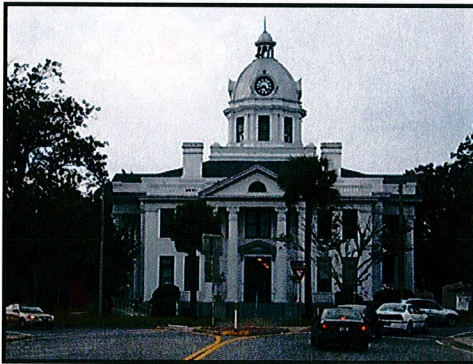
Untouched/Protected Areas: Jefferson County Courthouse Source: Jefferson County Studio
