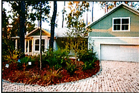
Permeable pavement increases recharge and reduces runoff. When combined with drought tolerant vegetation, stormwater is appropriately managed.
