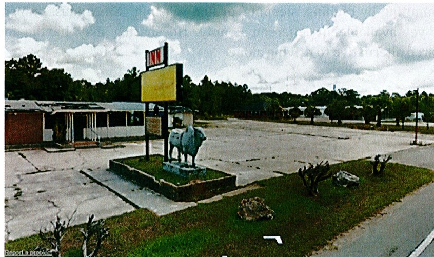
Potential park-and-ride lot off of US 90 at the Brahma hotel Source: Google Earth
