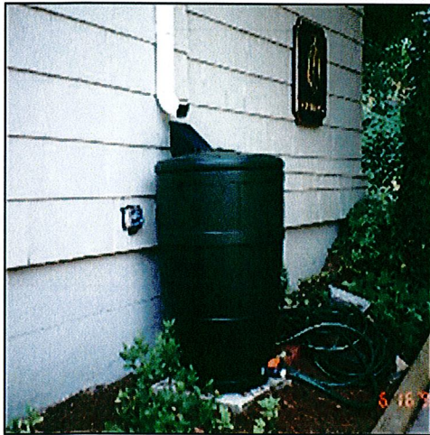
An example of runoff to a rain barrel, a way to catch and reuse stormwater. Source: Marty Wanielista, Stormwater Management Academy, University of Central Florida
